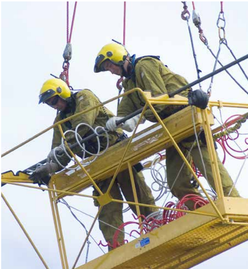
Two RTE linemen in the basket developed by their company for HEC missions.
